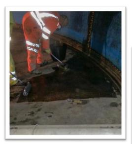
surface concrete repairs were carried out, before the prepared substrate was subject to the application of a Sikalastic Hot Sprayed Polyurea Waterproofing System, complete with a tack coat primer.
