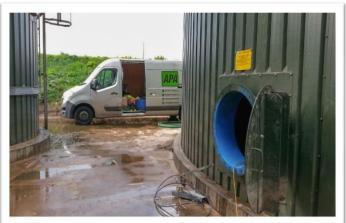
**The outcome:** The works within the primary digester tank were completed within a one-week period, ensuring the necessary remediation of the base cracking, with minimal disruption to the plant's daily activity. The choice of iron silicate propelled abrasive blasting allowed for surface cleaning without excessive particle breakdown, resultingly reducing the quantity of
